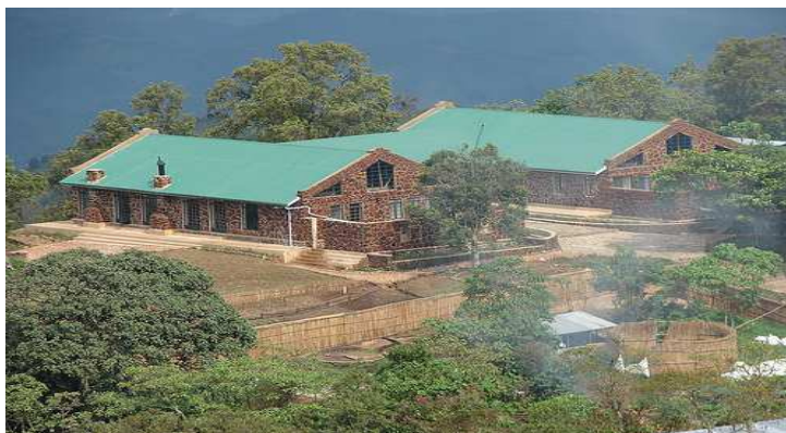
Figure 14: Acommunity lodge in Bwindi National Park
